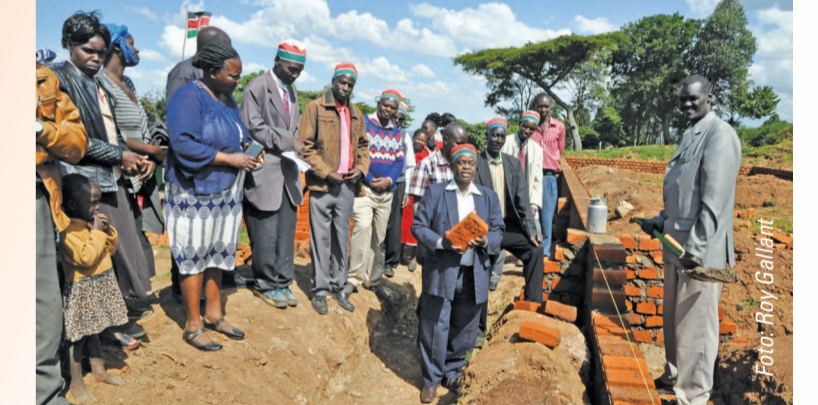
▲ Eerstesteenlegging schoolproject African Divine Church Kenia.
